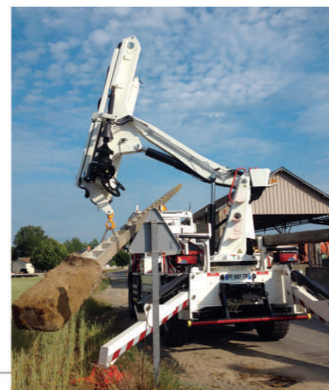
Drilling 100TA30 Stabilisation in A
